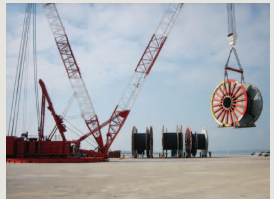
Crane at the jetty
