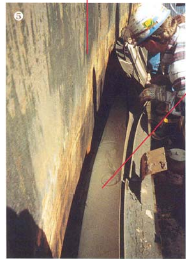
5 Time 3' 00" The foam delivered from each outlet meets up and blankets the entire seal area
