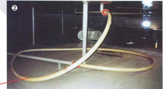
2 Time 0' 10" The foam is carried to a manifold on the roof through the COFLEXIP foam line, allowing correct delivery whatever the roof position.
