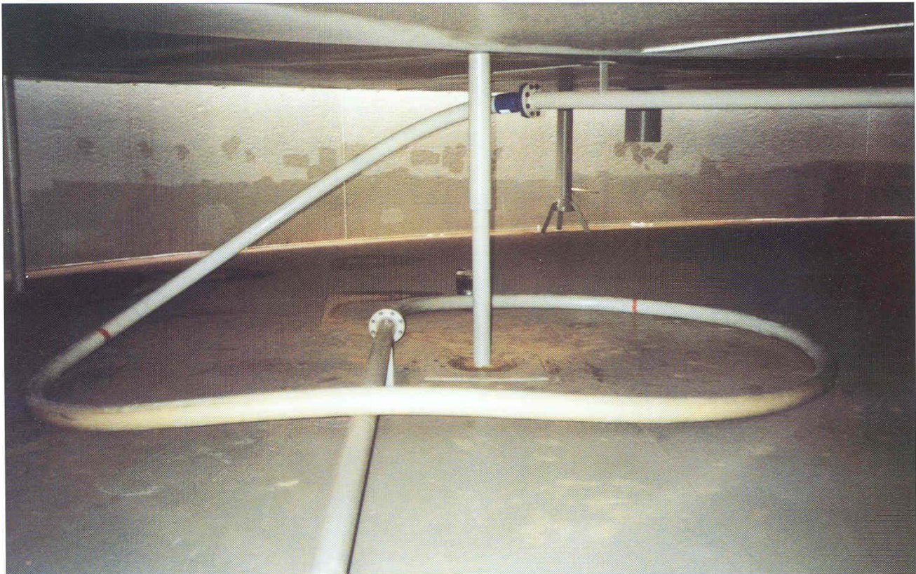
Installed Drain Pipe System
