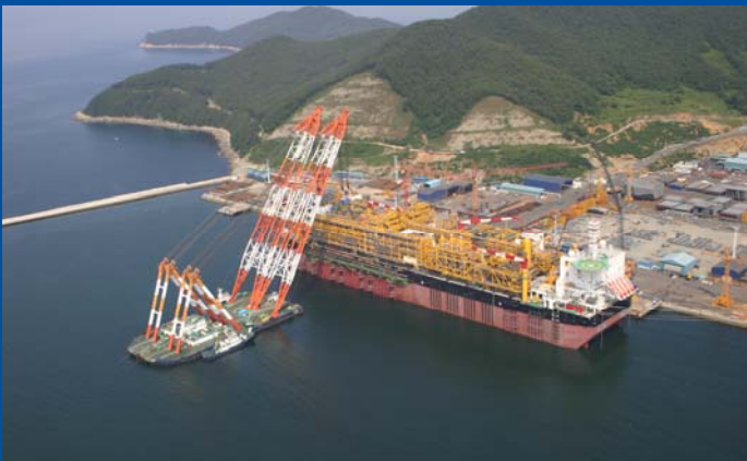
Total Dalia 28,000 tonne topsides 2003 - 2006
