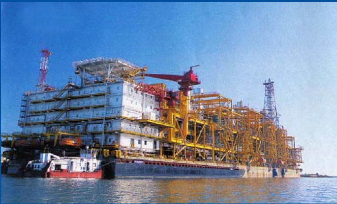
Elf Nkossa 30,000 tonne topsides 1992 - 1996
